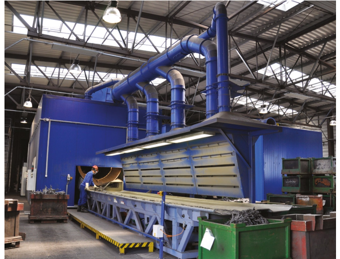
Knocking out castings and acoustic enclosures
