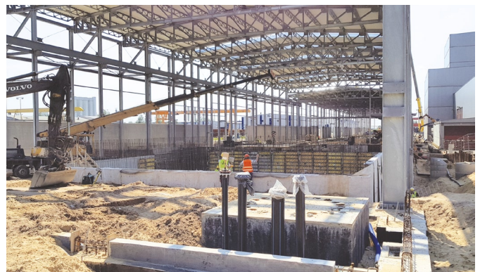
Building a new cast- iron foundry
