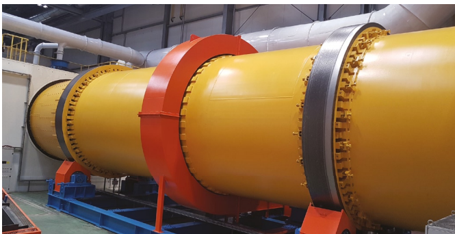
Installation of drum Q=300 t/h
