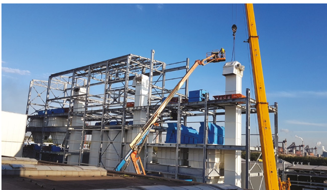
Installation of Sand Plant Q=300 t/h
